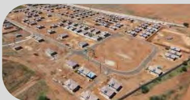
Mix Use Housing: Lethabong Housing Scheme
